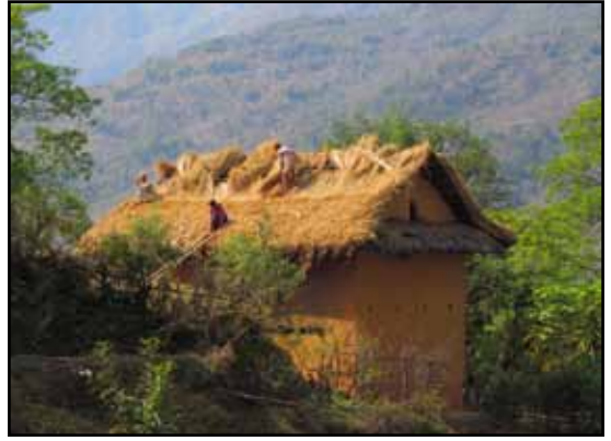
Day 7. Re-thatching a homestead barn in the hamlet of Chalise. The grass used for the thatching is the rice straw from the paddy fields after the harvest. In areas too high for rice to grow other grasses are used.
