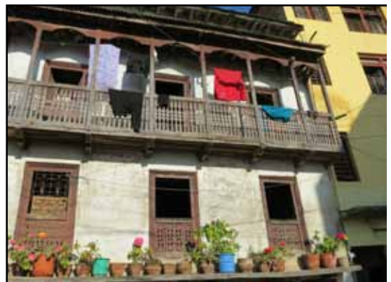
Day 13. The town of Gorkha is divided into an upper and lower half. The upper half is full of older houses and is generally free of traffic, while the lower half is newer and busier and is where most of the hotels are located
