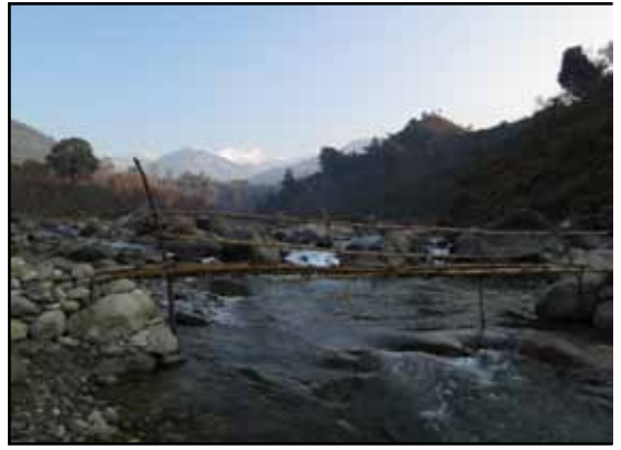
Day 16. Sometimes streams, and even rivers, are spanned with rickety bamboo bridges made with many stems lashed together. They are surprisingly strong but are usually temporary as the monsoon rains often wash them away in July or August
