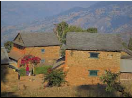
Day 11. Along the ridge to the north of the Kaste Khola are numerous hamlets of homesteads like this one at Ramichaur. Here the houses use large stone slates, dunga , as cladding but these are slowly being renewed with corrugated sheets
