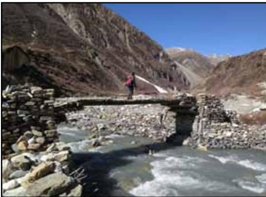
Day 12. Before the wire suspension bridges of the last 30 years all the bridges were of this cantilever type. Stones at each end anchored logs which protruded and narrowed the gap to be spanned.
