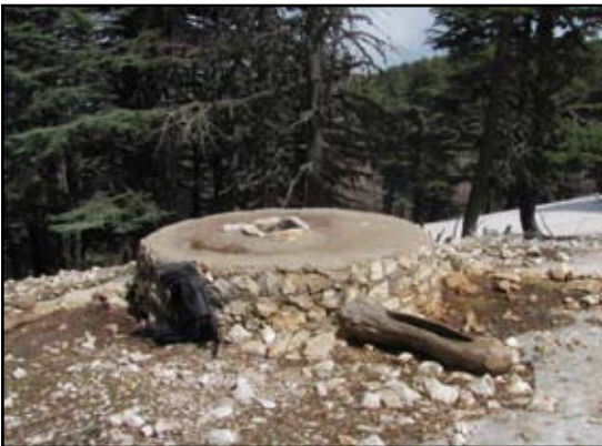
Day 18. A typical cistern where the surface water from rain and snow melt is channeled through the stone wall into a huge underwater tank where it is used in the summer months by pastoralists.
