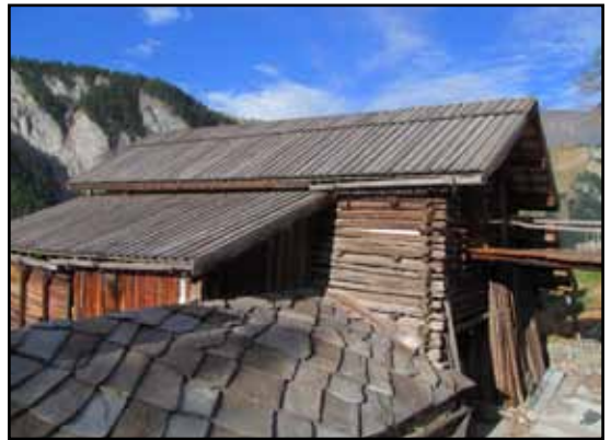
Day 1. The buildings of St Veran, and indeed throughout the Queyras region, are roofed in large slate stones or more commonly wooden planks. The walls are generally made of logs
